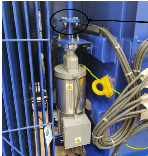
Breather pipe bottom flange fixing screws
